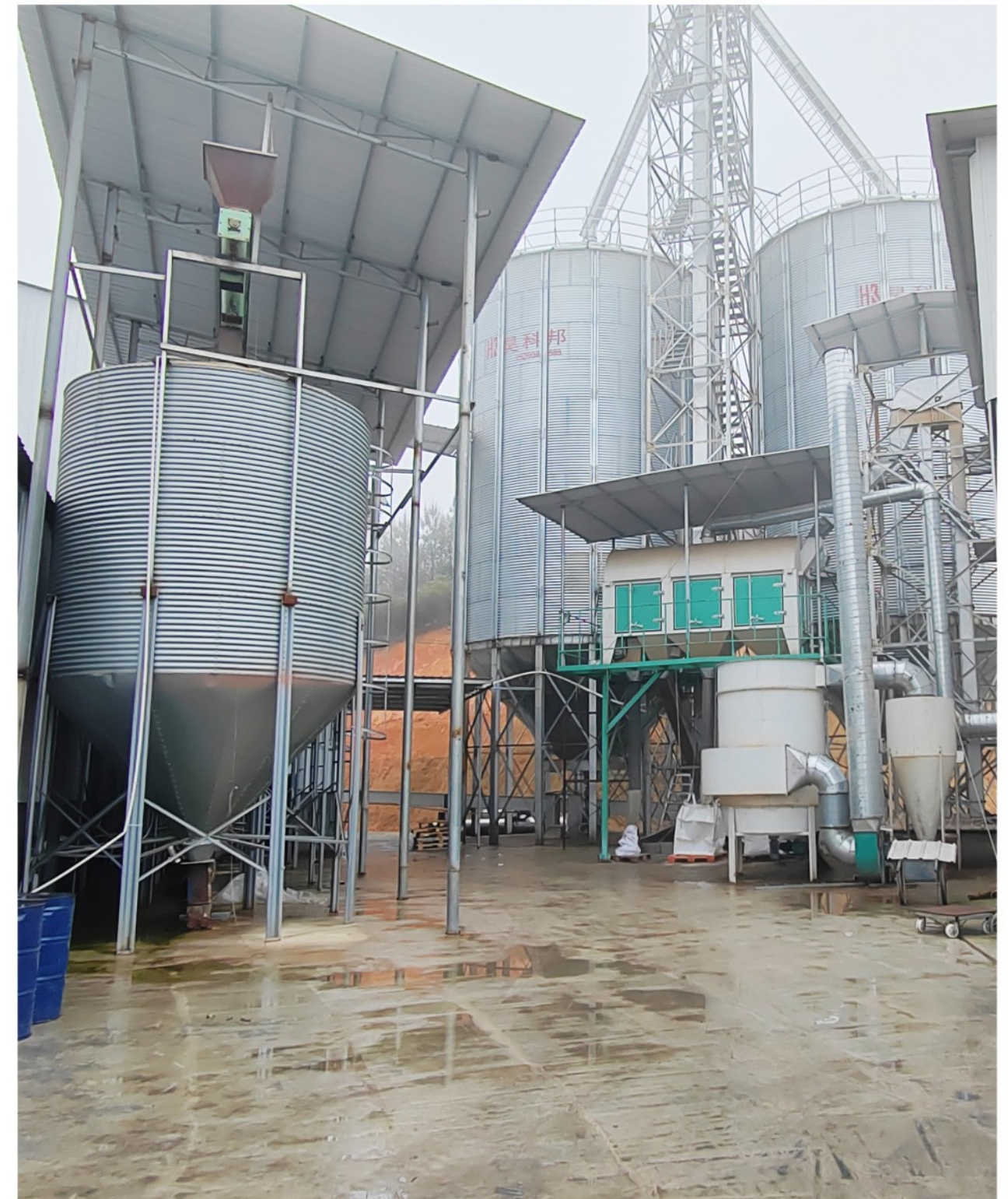
Pig Breeding Company Feed Silo Project
