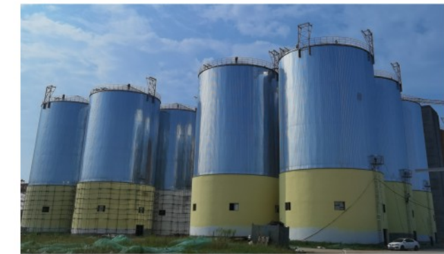
Cement cone bottom silo
