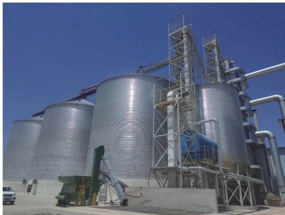
2020 Gansu Qingyang 5000T Cement Flat Bottom silo Project
