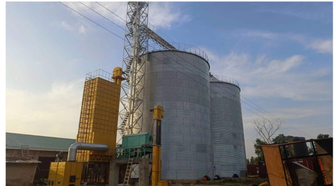
2023 Uganda 2-2000 ton flat bottom steel plate silo
