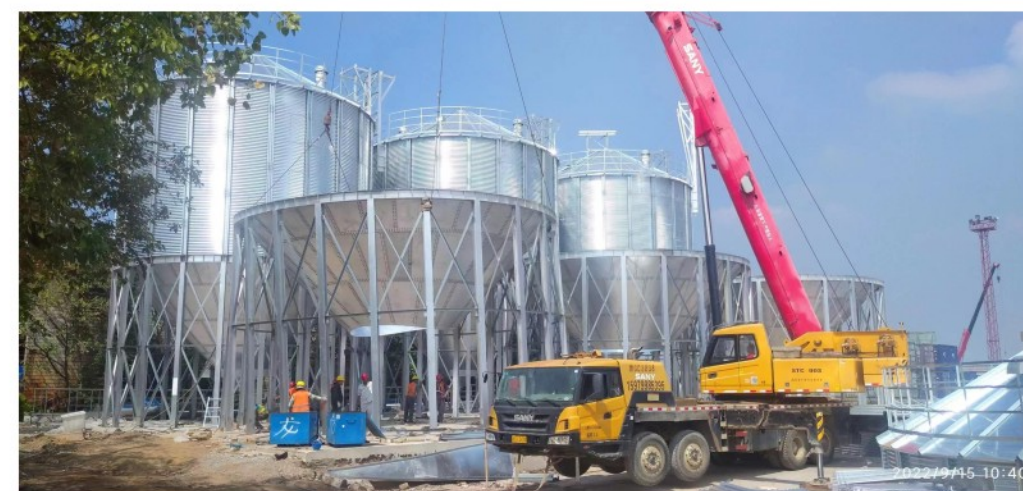
Jiangxi Jiujiang Shanggang Group Terminal Transfer Silo Project
