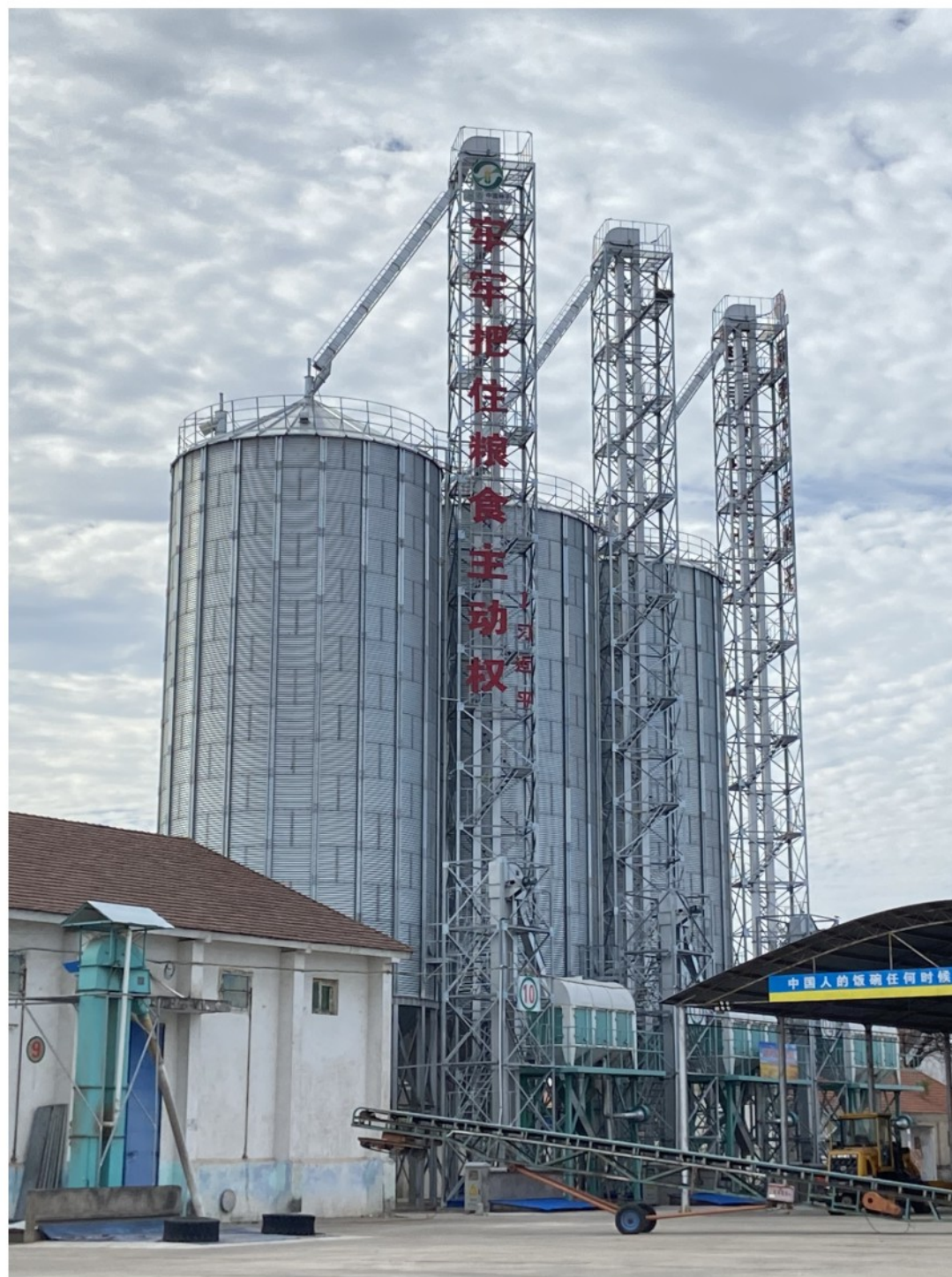
2021 Wen County Government Cooperation Project, 3-1000 Tons Conical Bottom Steel Plate silo
