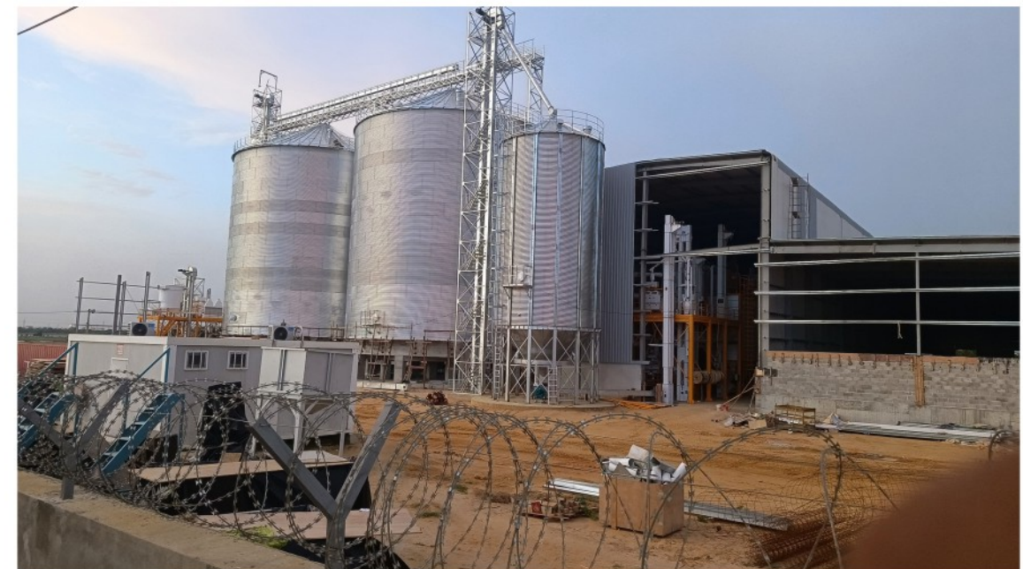
2023 Angola 2-4000 ton cement flat bottom silo+1-300 ton cone bottom steel plate silo
