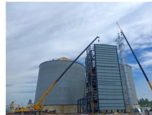
Cement flat bottom silo
